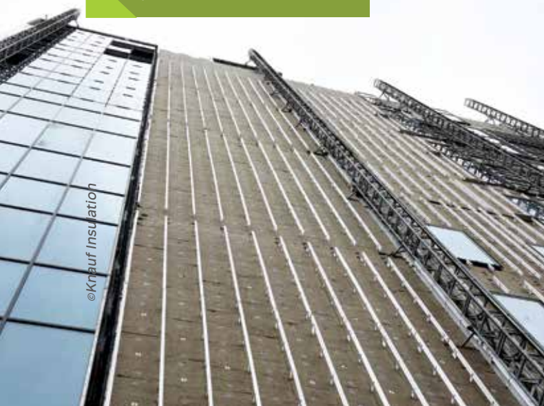
Typical External Wall Insulation
