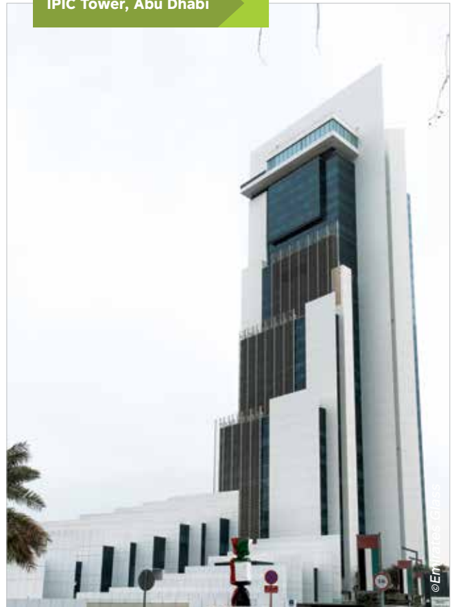
IPIC Tower, Abu Dhabi
