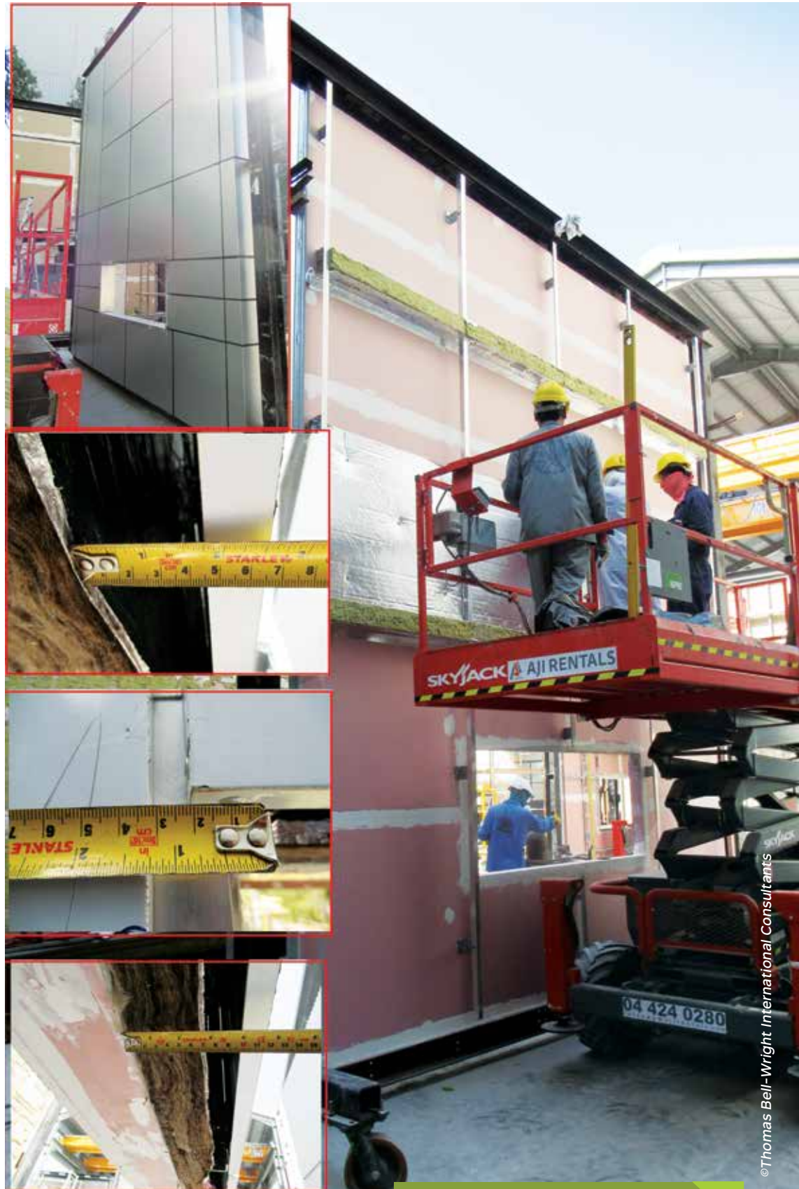
Figure 6: Installation in progress with insets showing details captured
