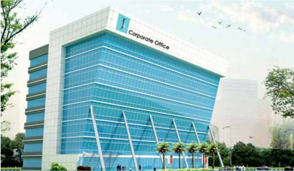
Jade 90, Mohali - was one of the initial projects in Punjab, which has a semi unitised glazing
