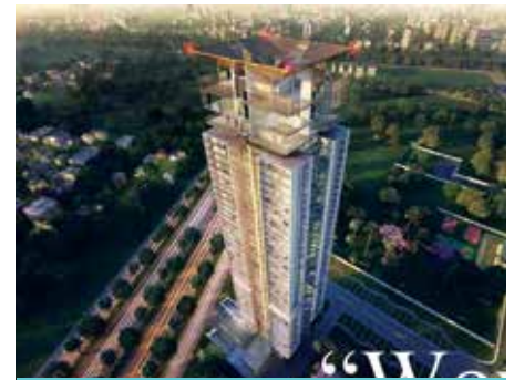
M3m Latitude - A skyscraper in the heart of Gurugram with high-end residences. The scope of work for Axsys was bespoke doors
