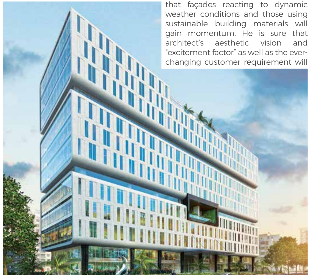
Aspee house -A commercial building at Malad, Mumbai. Resin with natural clay flexible tile cladding. By Vivek Bhole Architects Pvt. Ltd.
