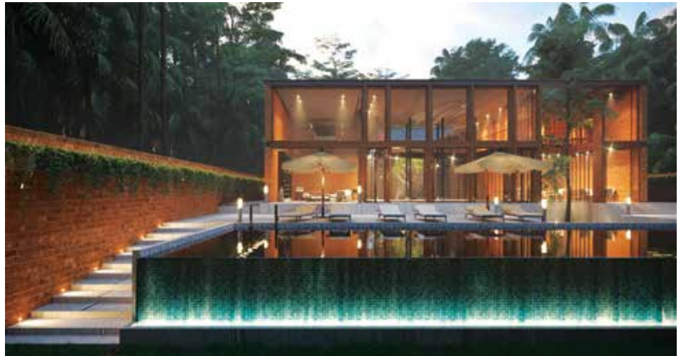
AIS Glass Villa - various kinds of glass used in its construction sets it apart
