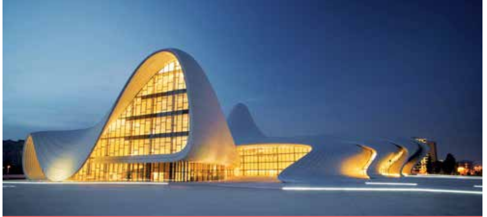
Heydar Aliyev Center, Azerbaijan: Glass fibre reinforced concrete (GFRC) and glass fibre reinforced polyester (GFRP) were chosen as ideal cladding materials, as they allow for the powerful plasticity of the building's design while responding to very different functional demands.
