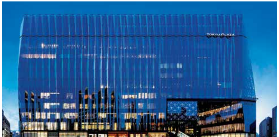
Tokyu Plaza Ginza, Seoul: The façade of this Tokyu Plaza Ginza Building consists of three dimensional glass planes, which creates a delicate phenomenon of light reflection and transmission. The unitized glass assembly is comprised of both low iron glass and heat reflective coated glass, treated with a 1mm ceramic dot pattern of gradient density.
