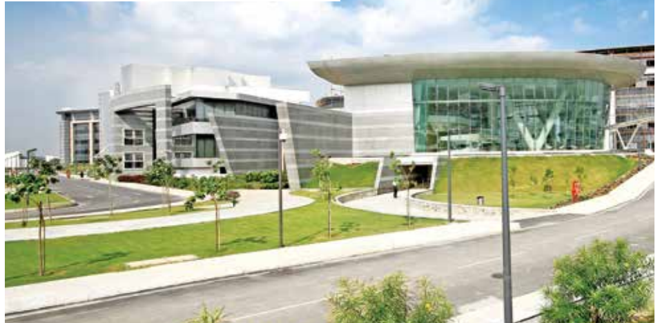
Syntel Global Development Centre in Chennai - The building footprint of each block assumed the shape of a pod with elliptical courtyards, into which the main office spaces open. Stone and glass were used in conjunction with aluminium composite Panels, to highlight the façade edges and form overhangs
