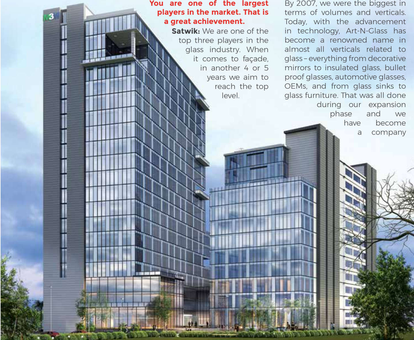
M3M Urbana - 6000 Sq m of unitised glazing, 2000 Sq m ACP, 2000 Sq m doors and windows
