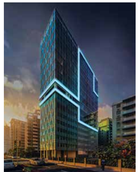
Tseries Studio cum commercial building of T-series super cassettes by Vivek Bhole Architects LED Lights with dichroic glass fin
