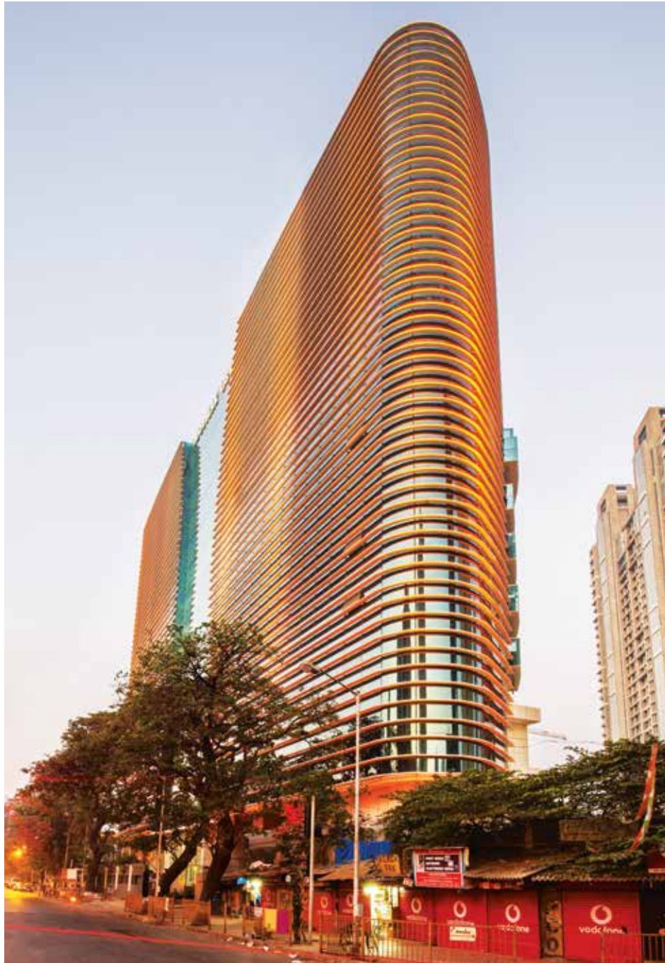
Another view of the Motilal Oswal building, Mumbai: Glass is combined with external shading elements to be able to perform at their peak level
