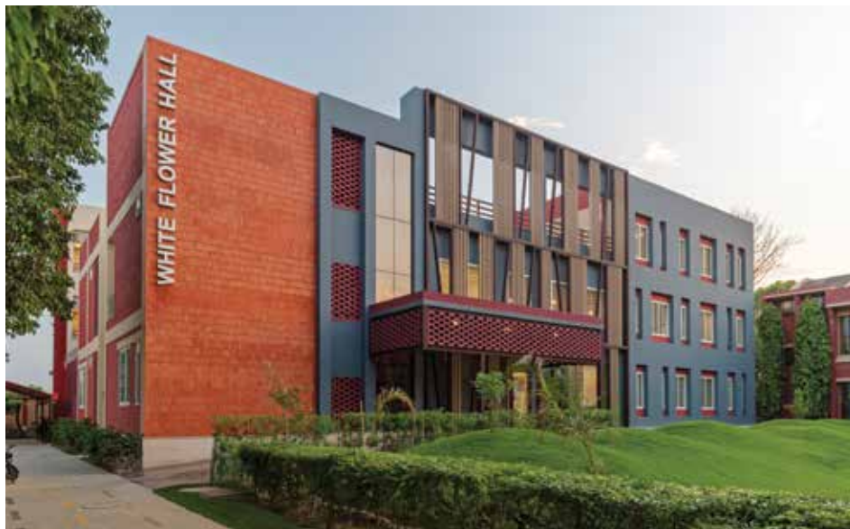
Overall view of the Girls Hostel at Mann School
