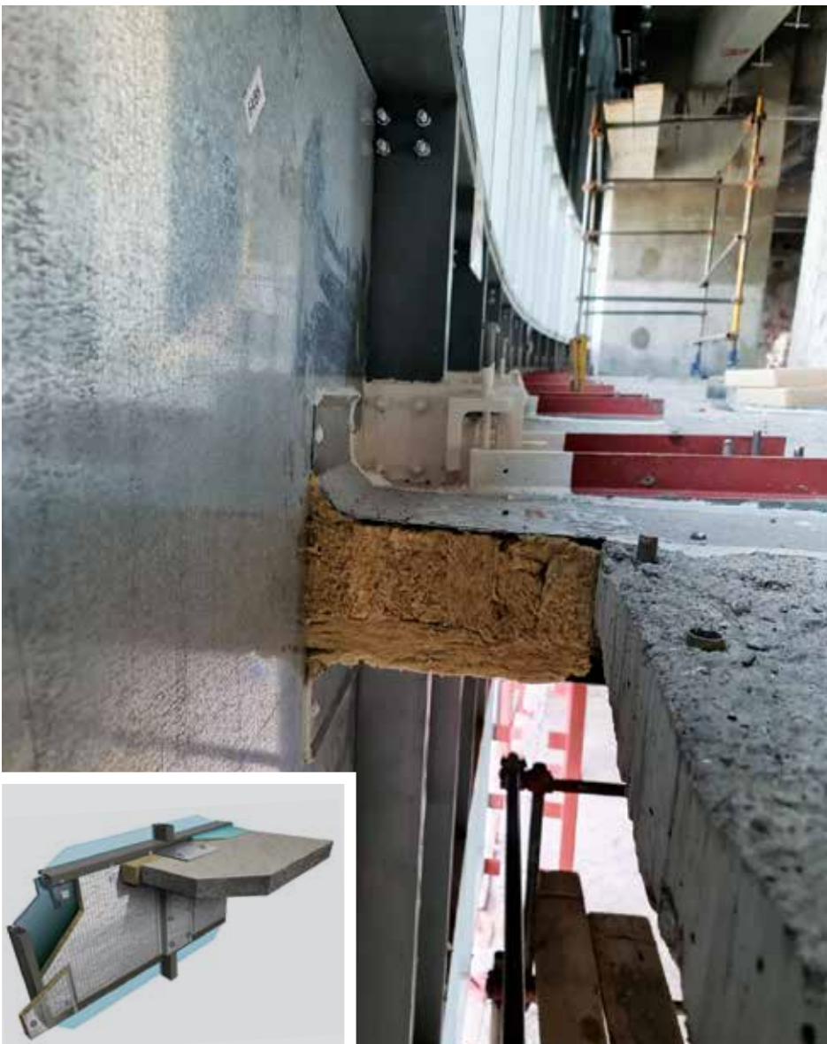
The void between a curtain wall and floor assembly being closed with fire stops
