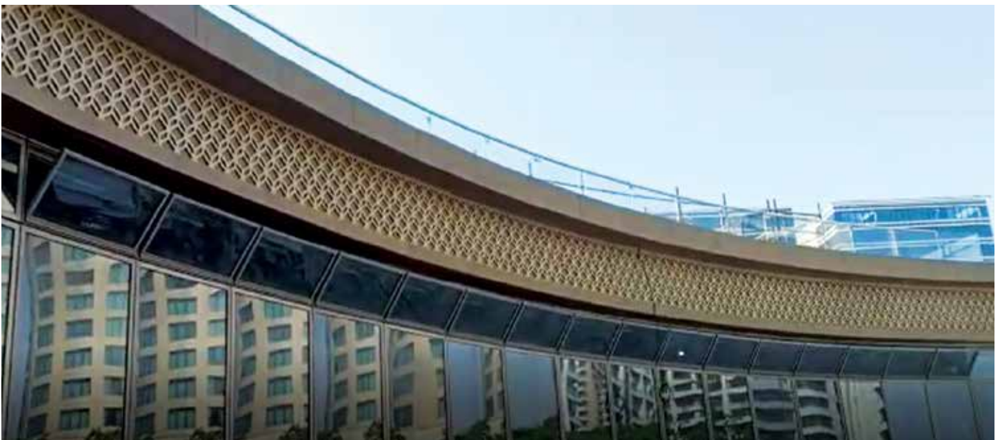
Automatic Smoke Ventilation Systems
