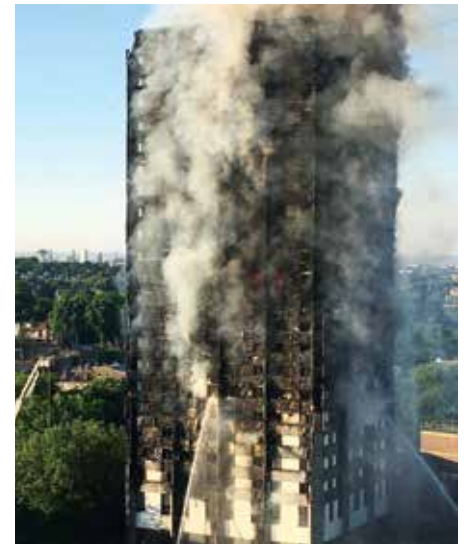
Grenfell Tower, UK - 14 th June, 2017 – Residential building.
