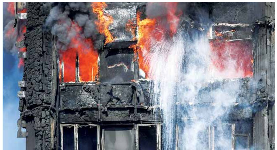
Damage to the face of the building – Grenfell Tower, London
