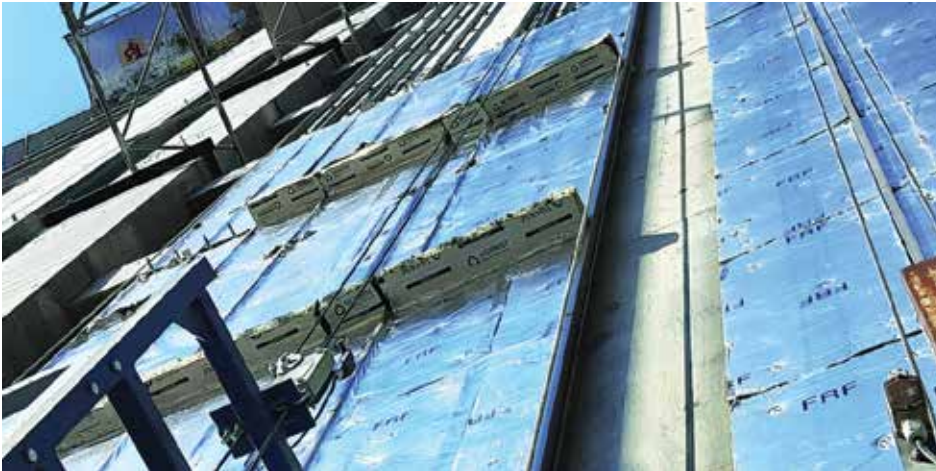
Siderise CH-CB Closed State Horizontal Cavity Barriers in conjunction with RV Rainscreen Vertical Cavity Barriers provide effective compartmentation
