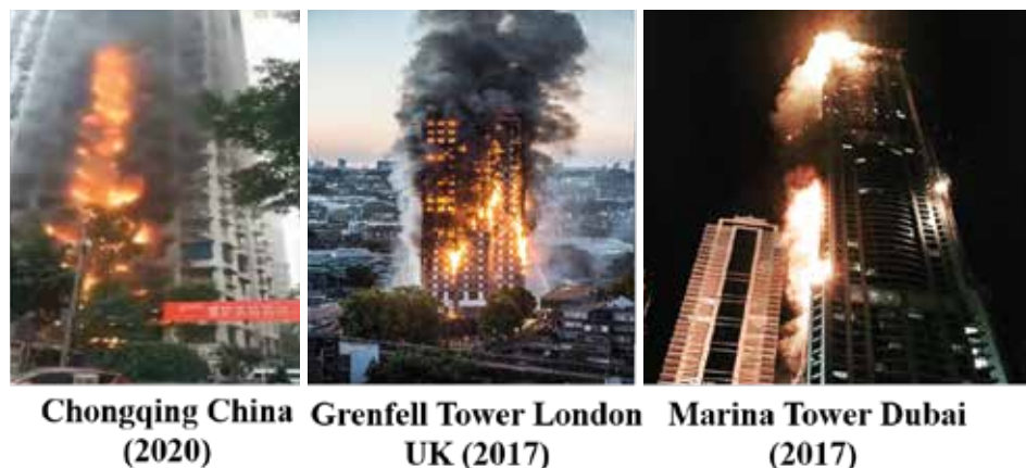
Figure 2: Recent high-rise building fire accidents
