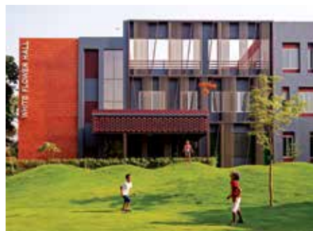
The front façade of the Girls Hostel at Mann School has a play of brick and metal jaalis
