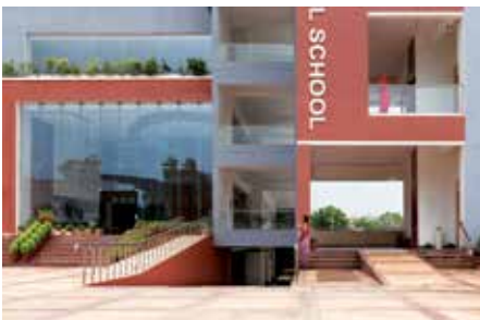
Another view of the façade with the entry to the basement
