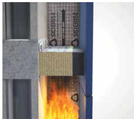
In the event of a fire, the intumescent material on open-state cavity barriers expands in reaction to high heat
