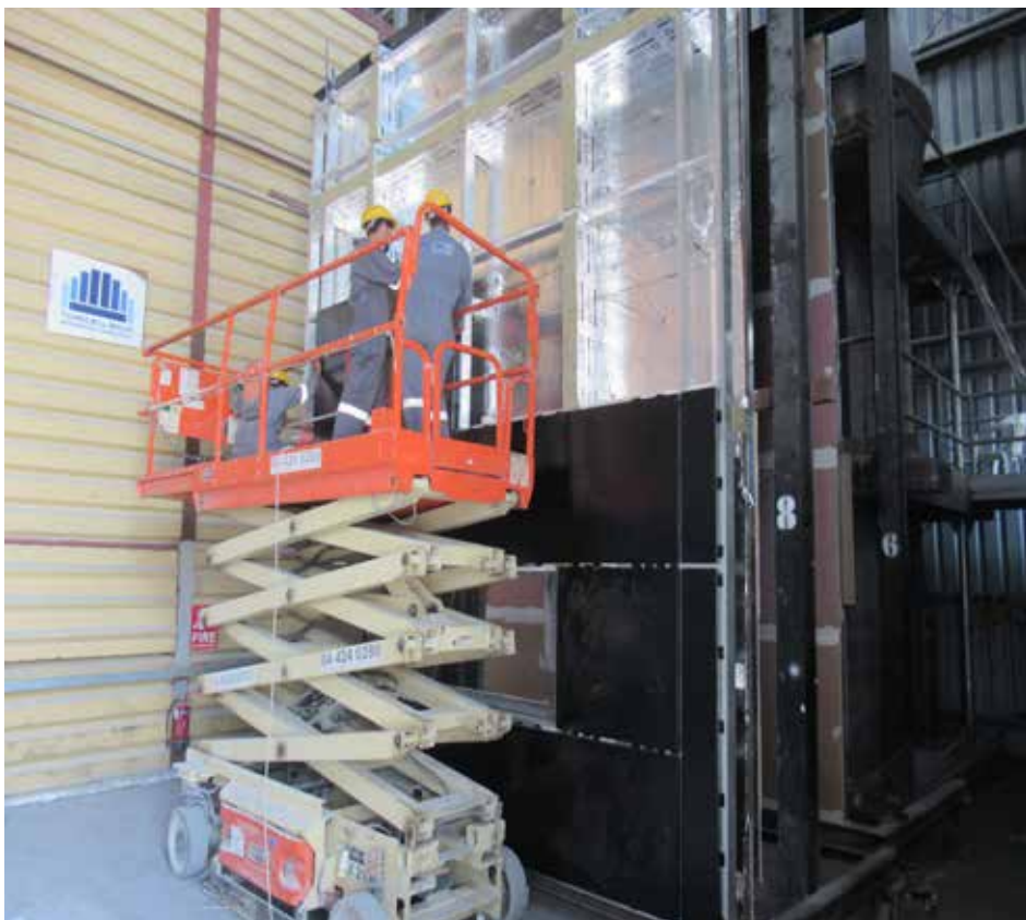
Picture 1: A mock-up is getting built up for a test to be conducted as per the NFPA 285 test method
