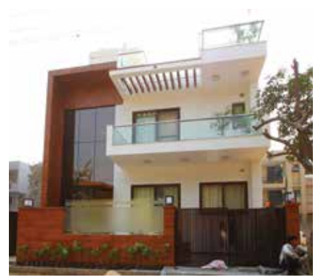
Façade treatment for Anand Villa in New Delhi
