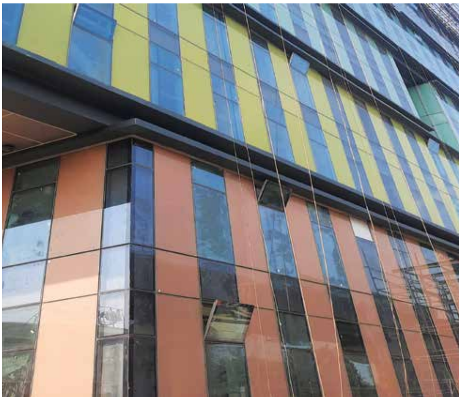
The smoke ventilation system in a School-K12 International in Kolkata
