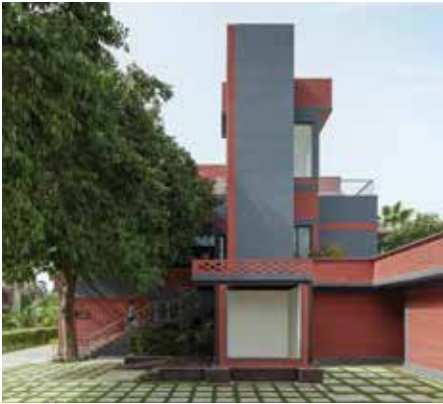
Brick façade of the Director's Chambers at Mann School, Delhi
